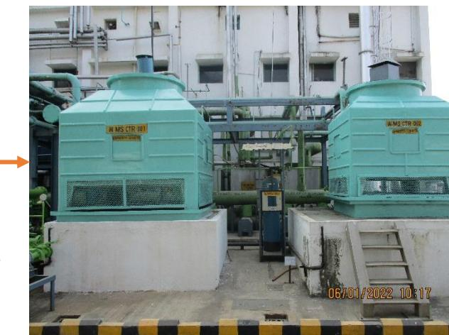
All the Treated water from RO & Evaporator is used for cooling tower make up (Recycle & Reuse)
