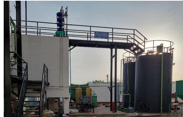
After Primary, Secondary & Tertiary Treatment, ETI Treated water feeds to Reverse Osmosis (RO) Plant.
