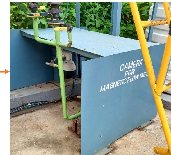
The Treated Water from RO (RO Permeate) is transferred through Magnetic Flow Meter where OCEMS Camera is installed.
